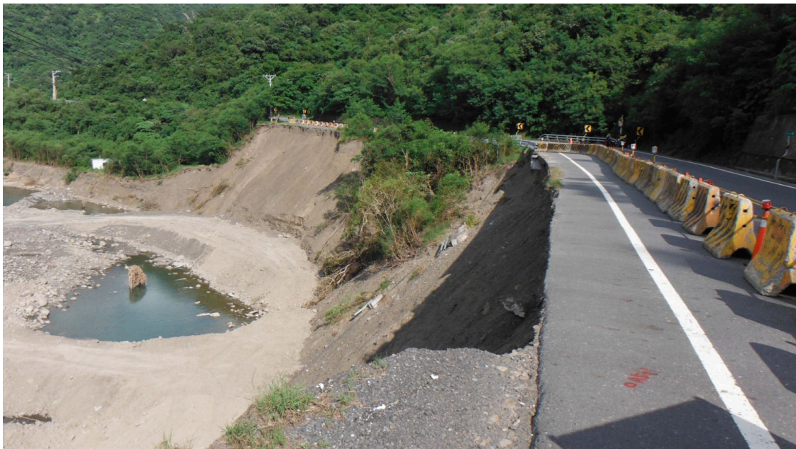
Figure 2. Severe scouring smashed the riverbank and caused disruption of the highway.
