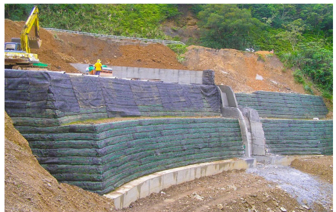
(b) Construction of reinforced earth slope.
