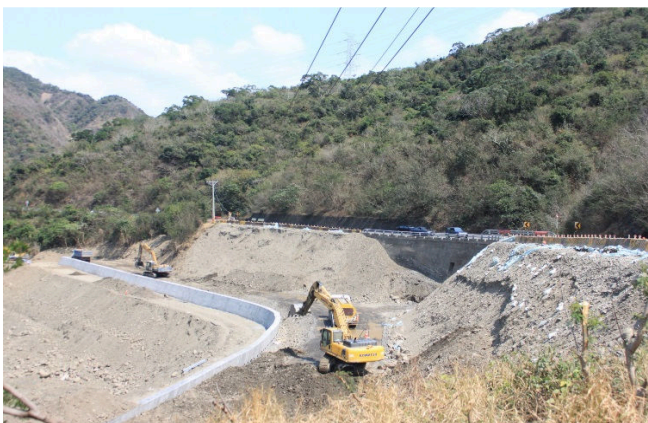
(a) Construction of pile-supported protection wall.
